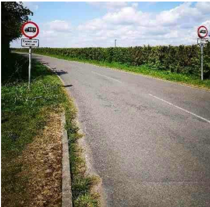
Figure 2-5: High Ditch Road- Site Visit
